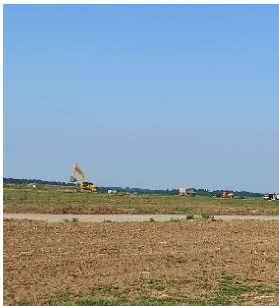
Figure 50: Final removal of vegetation
