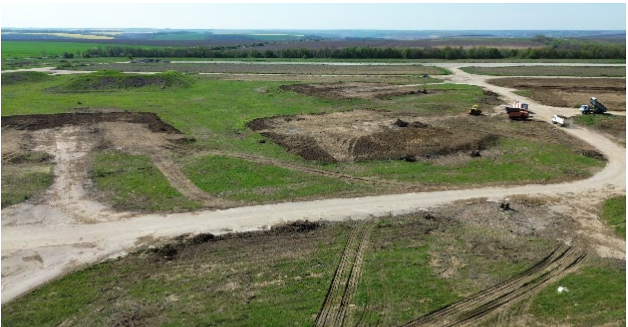
Figure 69: St. George site during the earthworks
