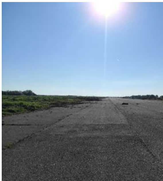
Figure 48: Airport runway (post clearance) (May 2023)
