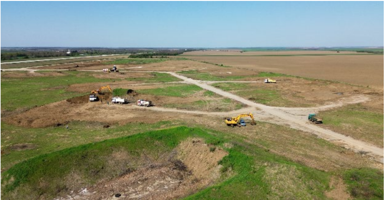
Figure 68: St. George site during the earth works
